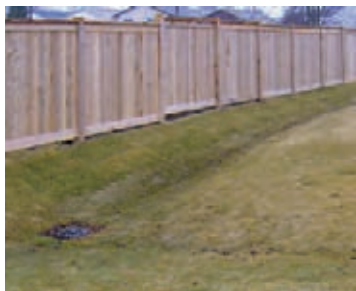
Typical backyard swale with a drain.
